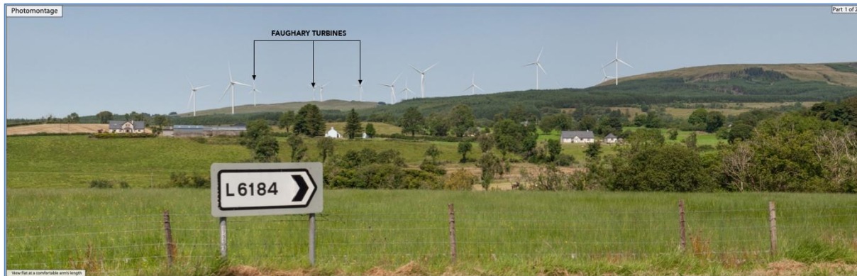
Figure 13-18: Assimilation of existing Faughary turbines within the proposed turbine array
